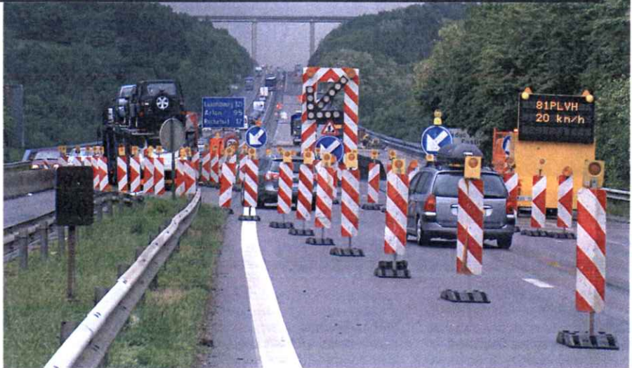
↑ Mobile ANPR linked to portable VMS can be a valuable warning system for areas such as work zones
